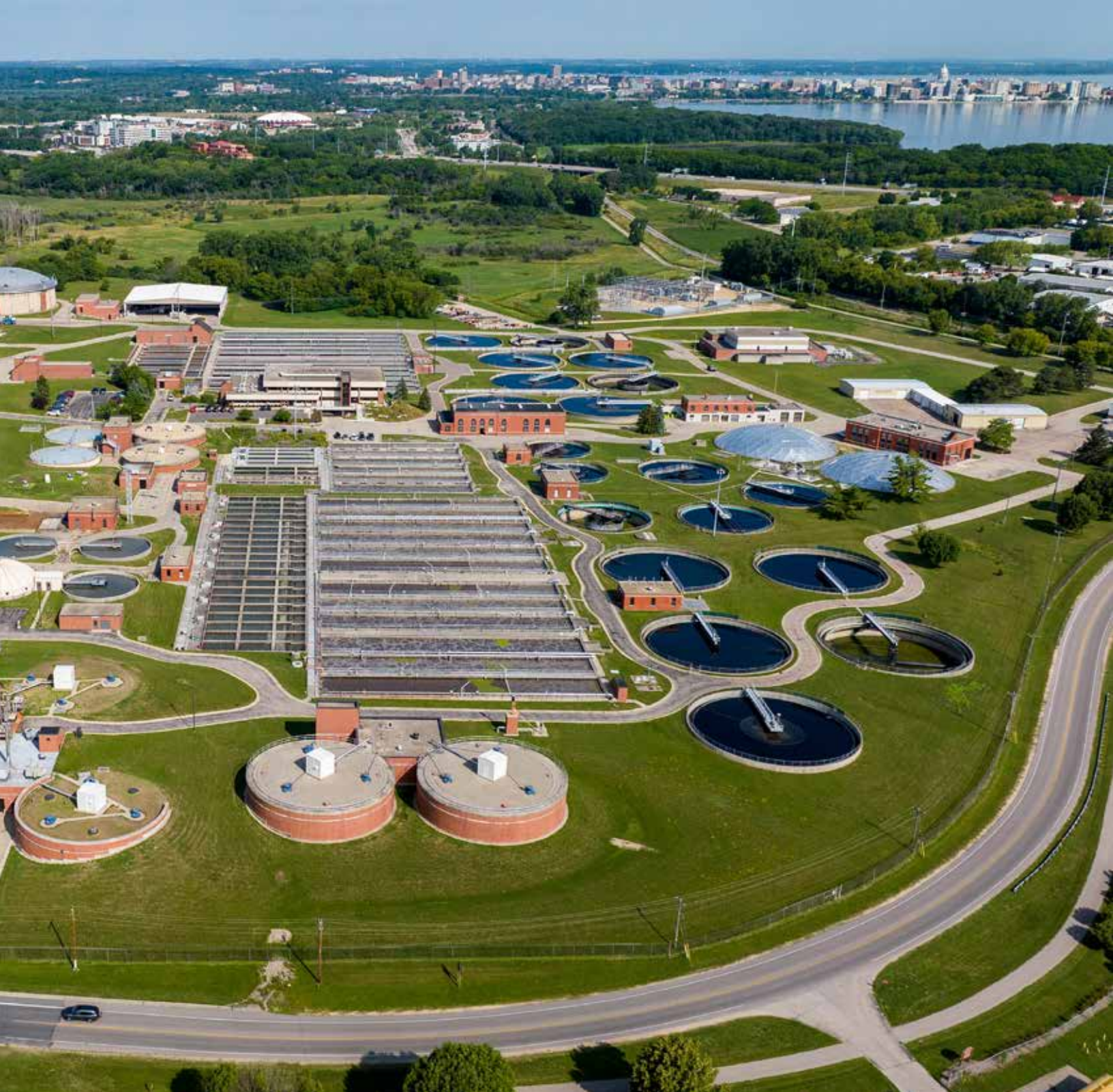
An aerial view of the Nine Springs Wastewater Treatment Plant.
