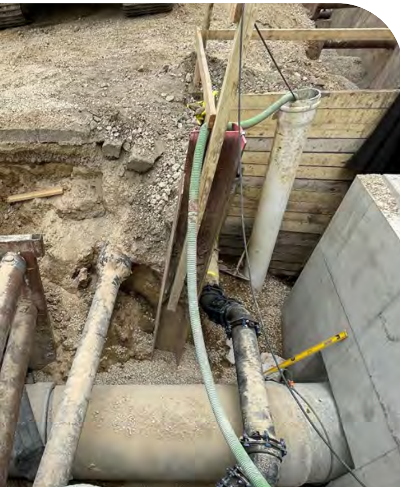
The 2023 repair of the West Interceptor at Marshall Park on Allen Boulevard required repairs to 60 feet of 30" pipe and three structures.
