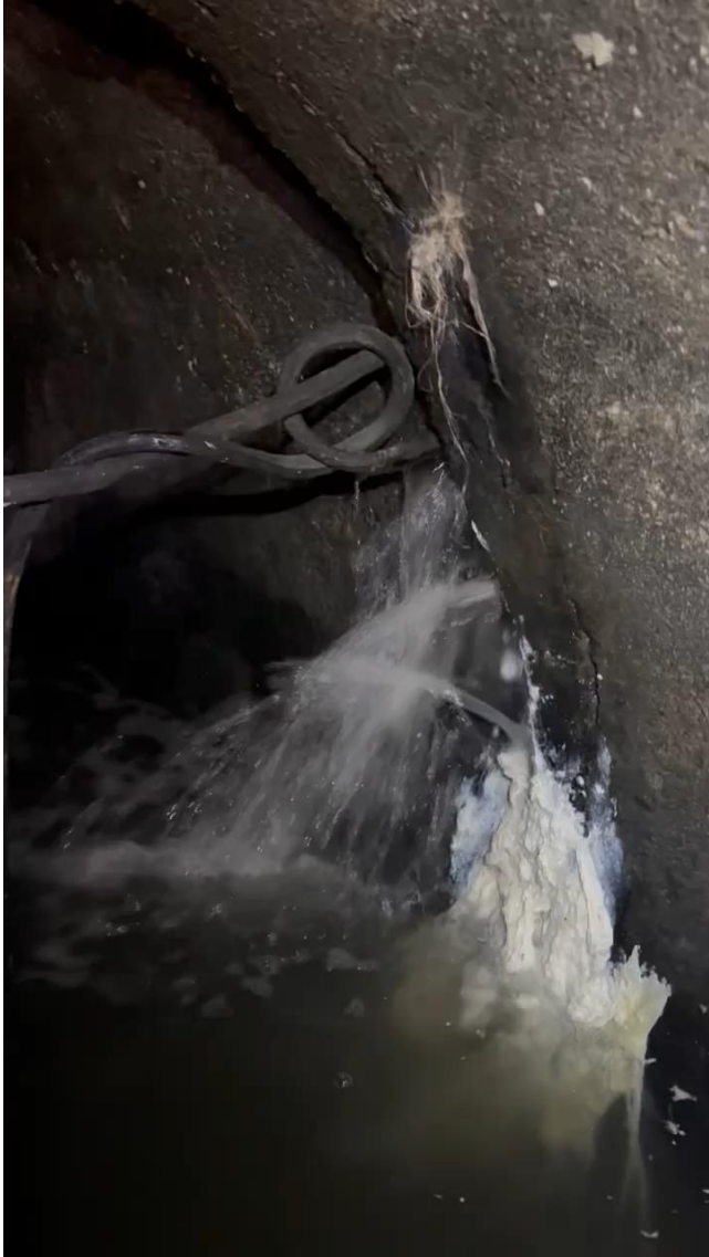
Video: Offset Joint during repair
