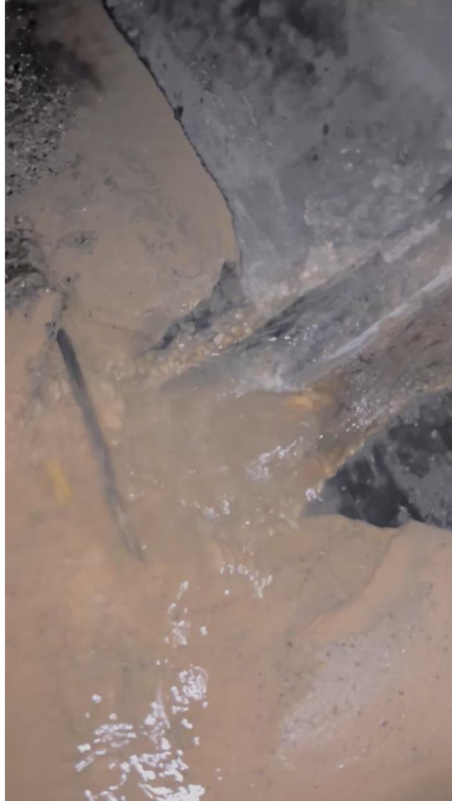
Video: Offset Joint during repair
