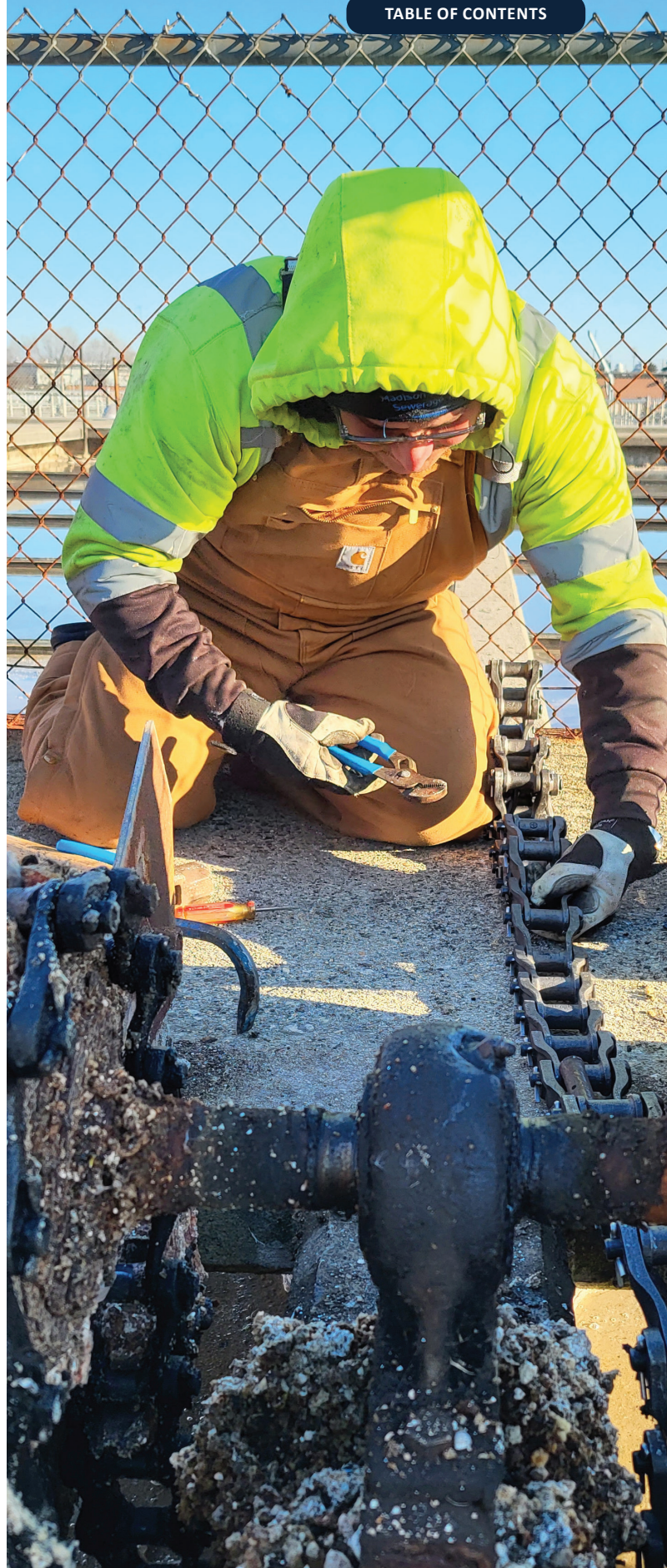
Mechanic Rigoberto Ramon-Solis works on a primary tank drive chain in the cold of winter.
