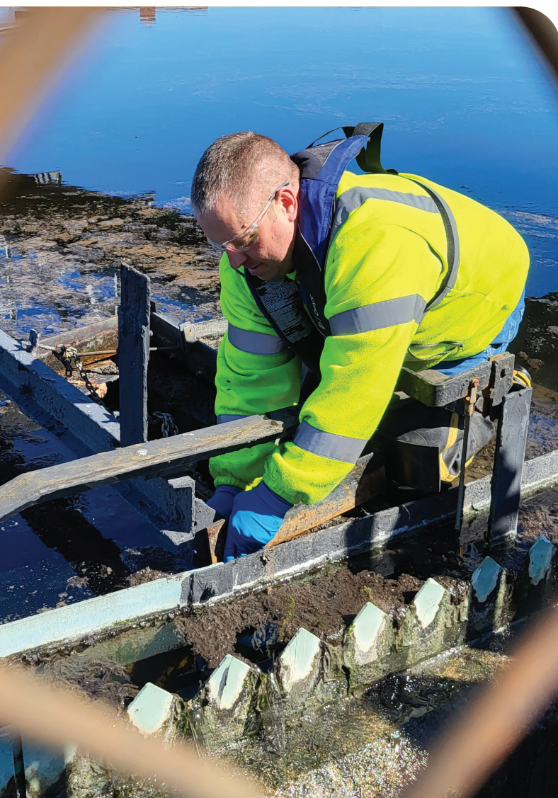
Facilities maintenance technician Chris Lothe repairs rubber on a final clarifier sweep arm while positioned on the scum beach.
