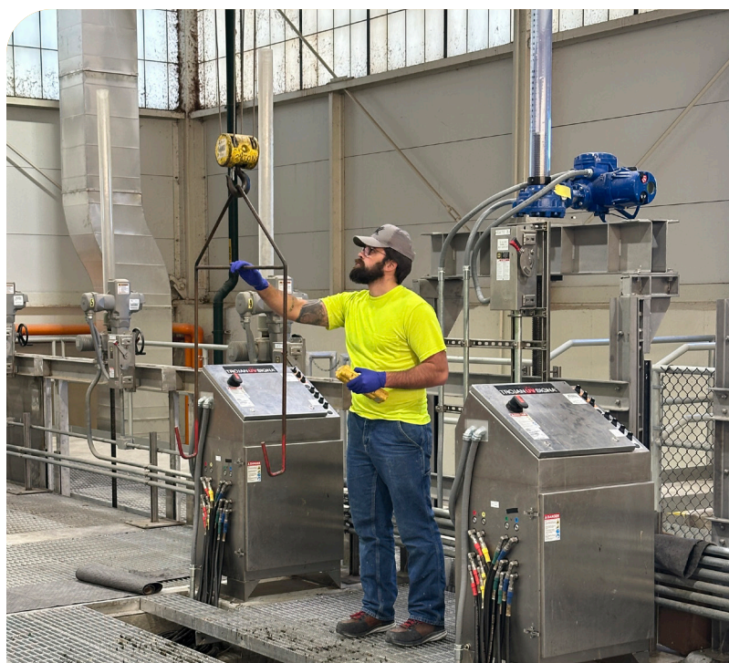
Operator Mitch Koller prepares to raise the UV screens in the Effluent Building for manual cleaning and removal of filamentous algae.
