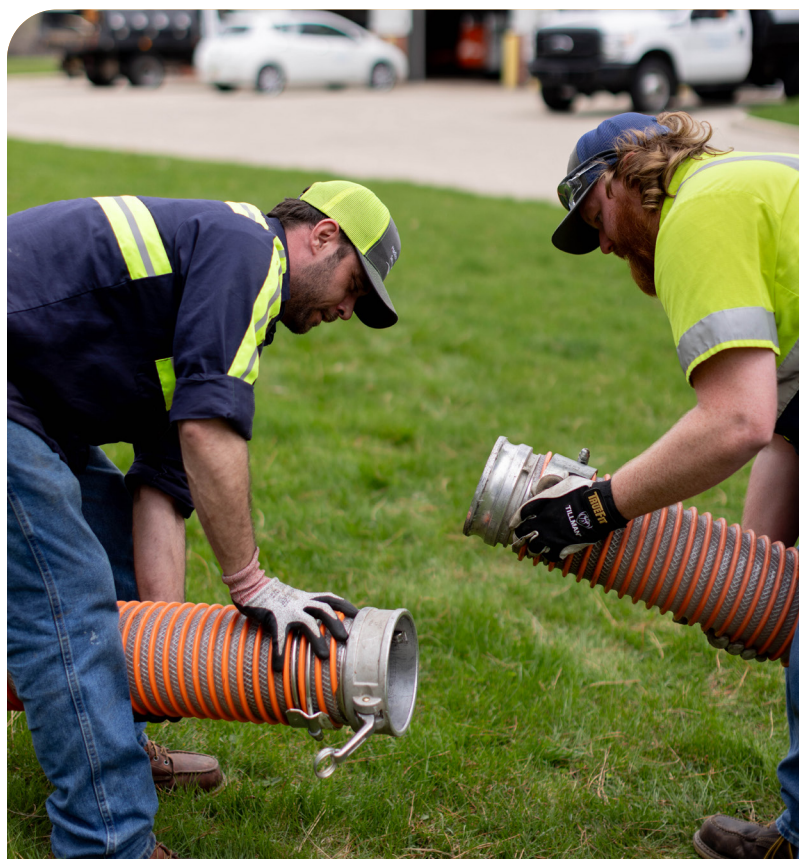
Facilities Maintenance staffers Justin Boyd and James Dinges connect industrial hose at the Nine Springs treatment plant.
