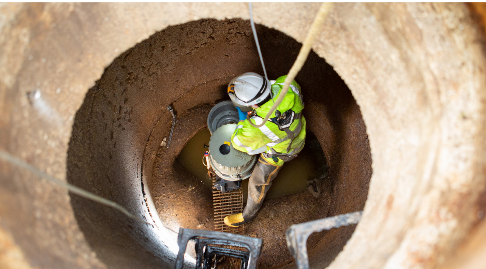
Collection System Services worker at the District, collects samples and flow data from inside a manhole.
