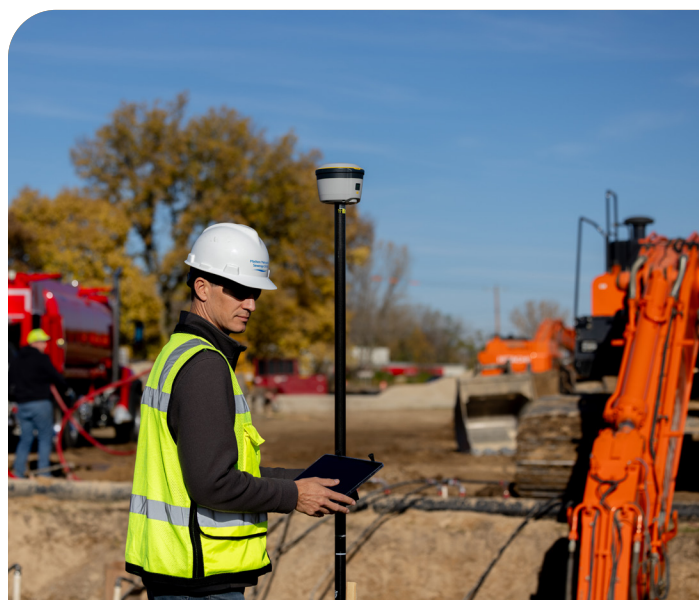
Project Engineer Aaron McFarlin uses a locator pole at the NEI-Waunakee Extension construction site.
