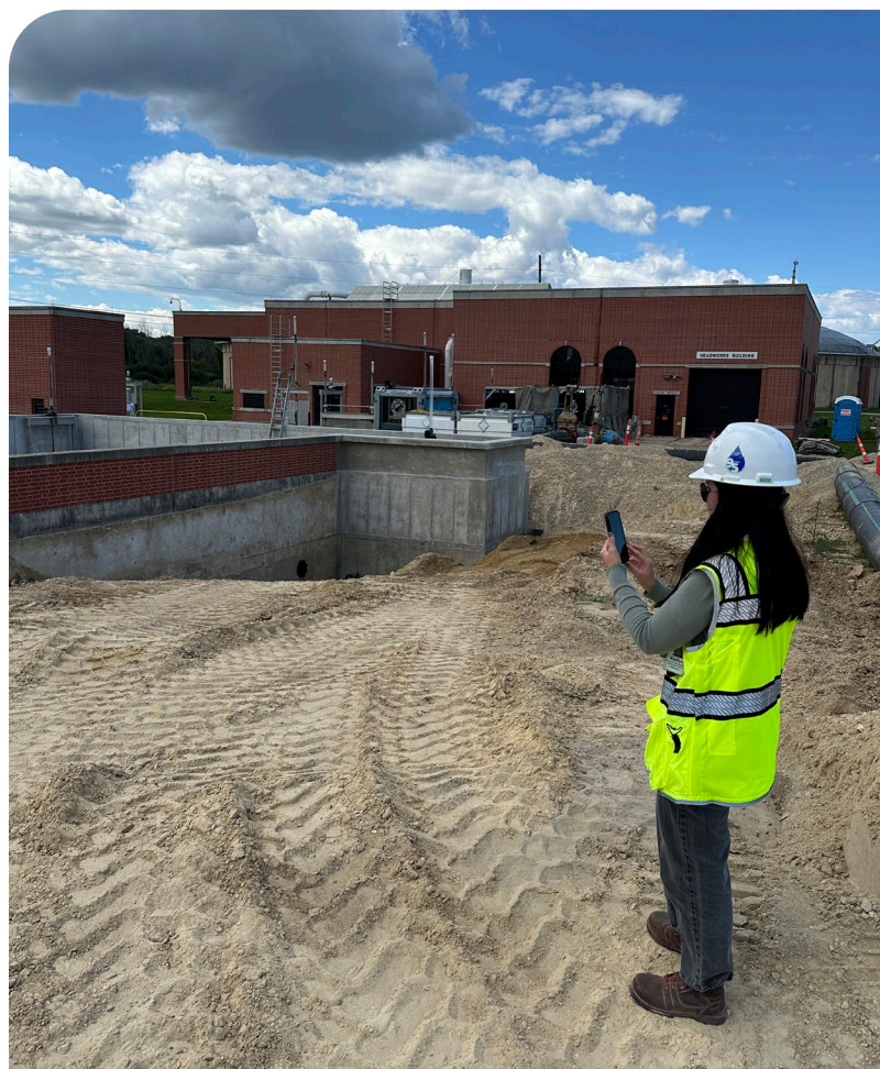
Project Engineer Kaylin Hackeloer-King inspects progress on the Flow Splitter Improvements project.
