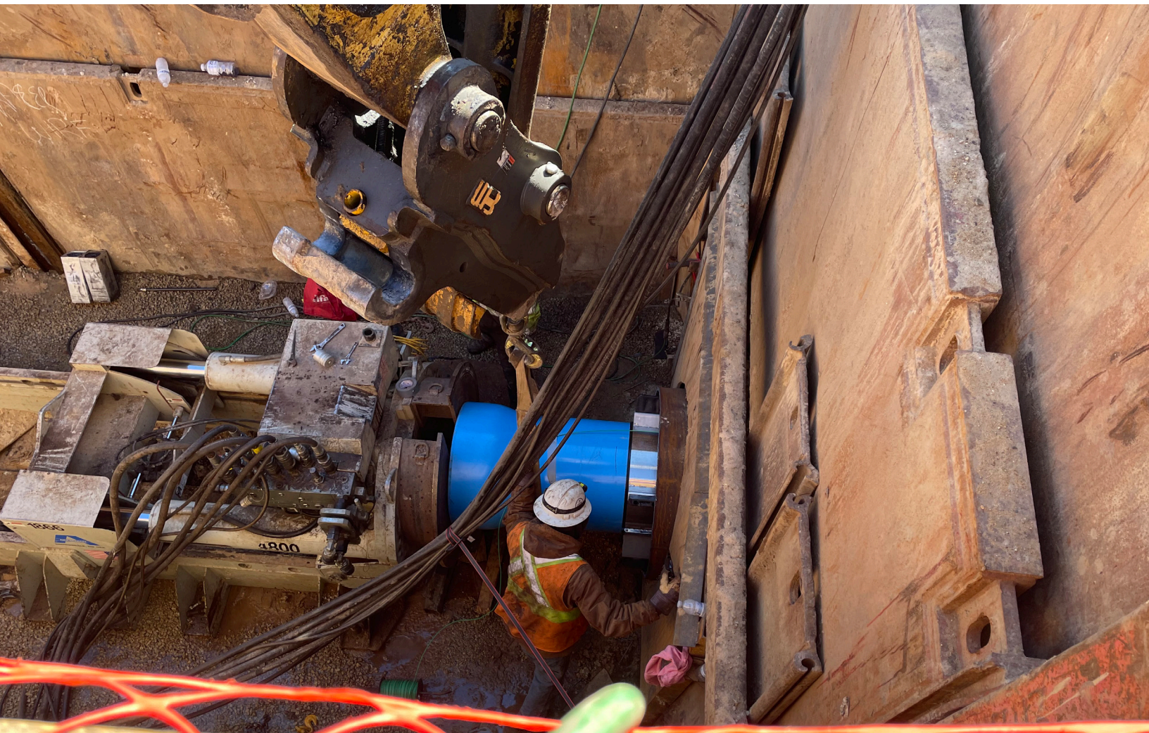
A crew installs a 24-inch sanitary sewer pipe in a 42-inch steel casing pipe on Pumping Station 17 Force Main Relief - Phase 2 project. This pipe was constructed by trenchless technologies under Old Highway PB in the Town of Verona.
