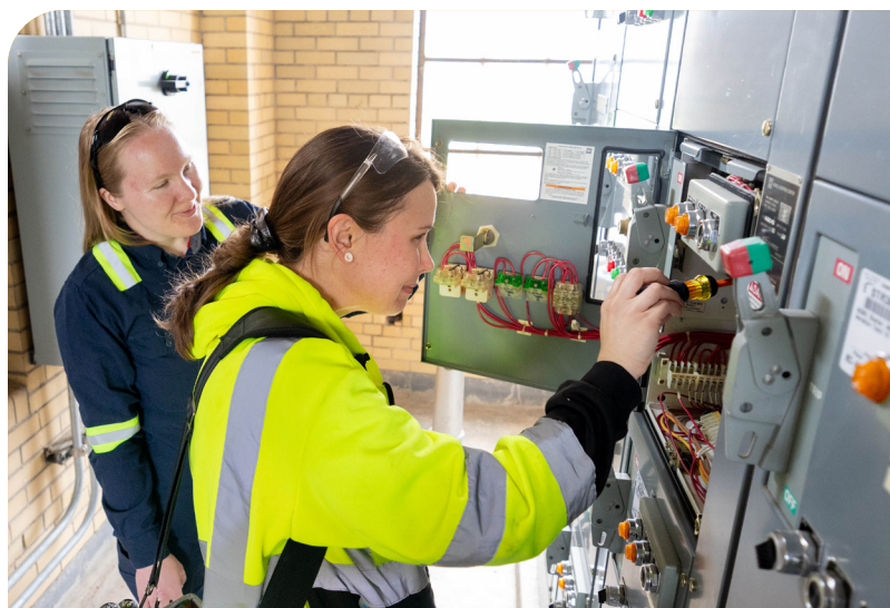
Apprentice electricians Taylor Cross and Anna Wright perform preventive maintenance on electrical equipment.
