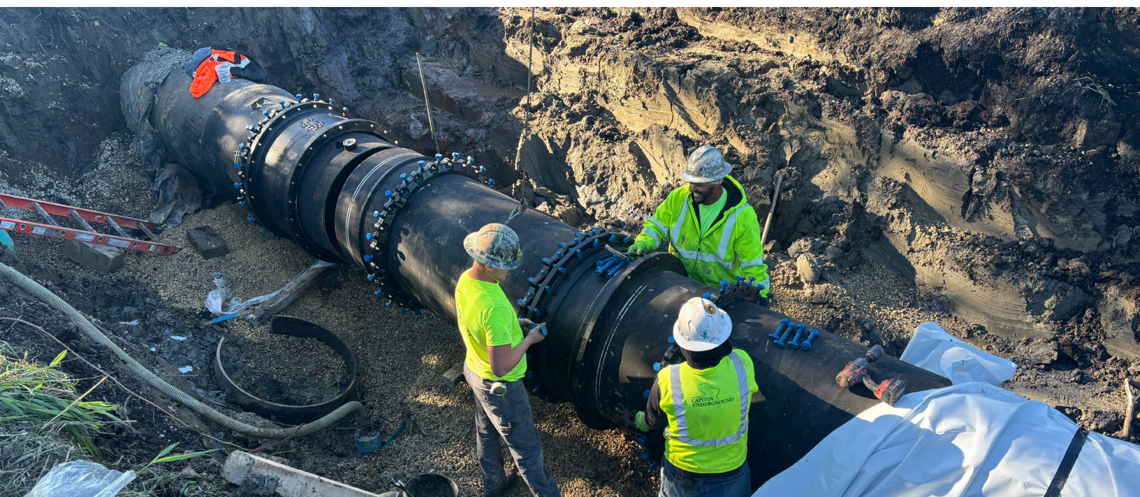
Contractors work on the final repair of the Pumping Station 2 Force Main following an August 2025 sanitary sewer overflow.
